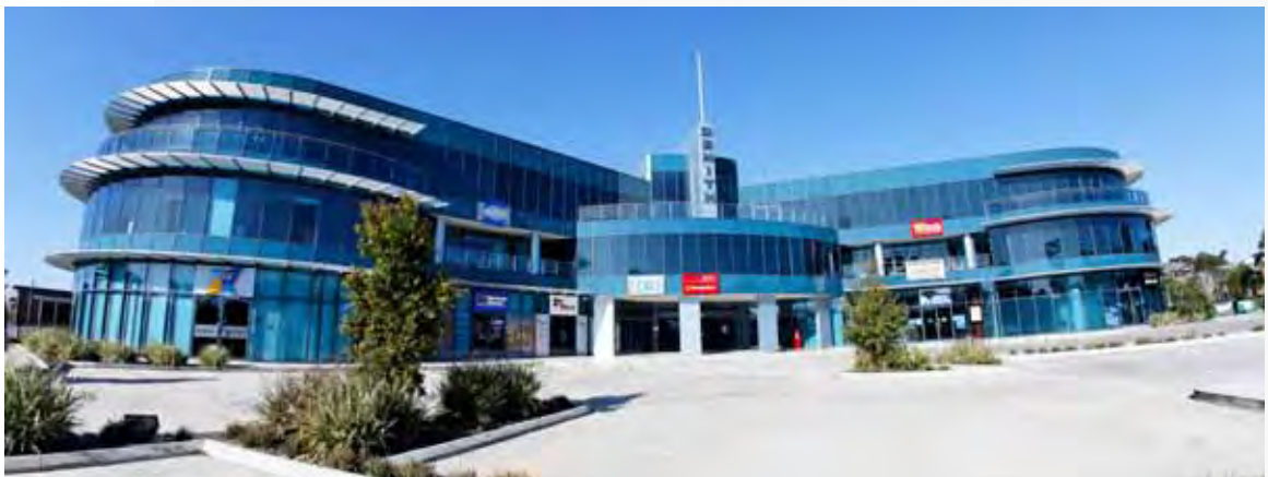
Zenith building, Tuggerah Business Park.
