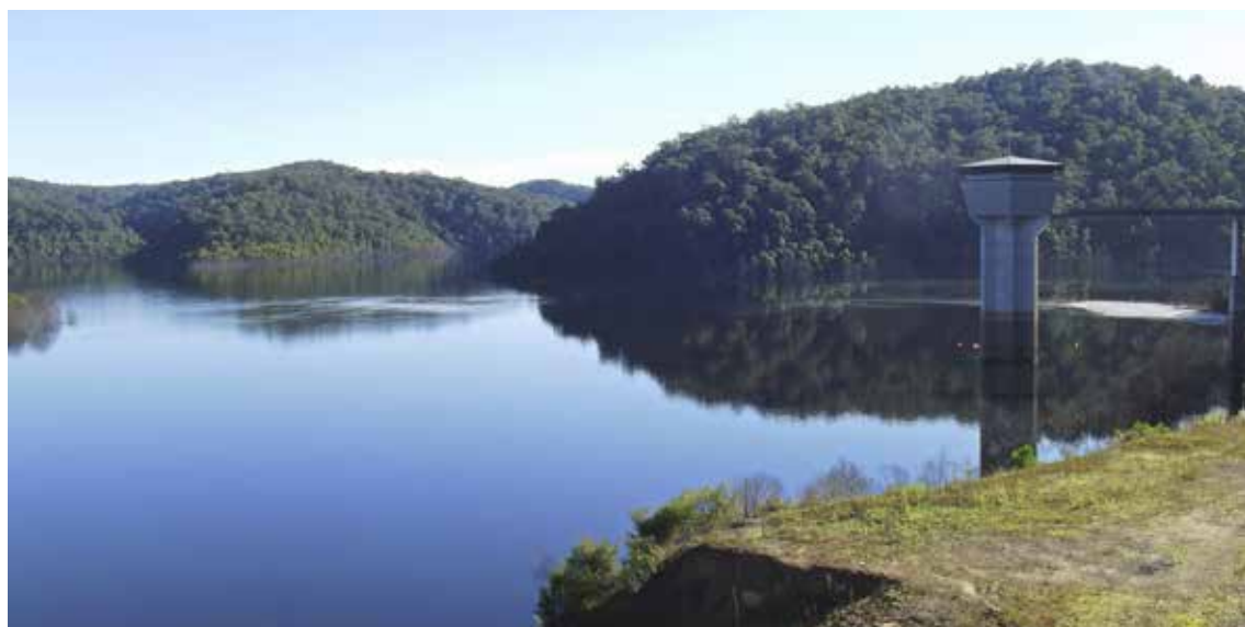
MANGROVE CREEK DAM
