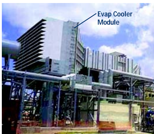
Donaldson's Evaporative Cooler fits neatly behind any of the Donaldson air inlet filters -- in this case it's downstream of a GDX self-cleaning filter.
